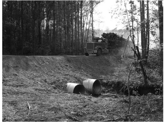
**Figure 5. Culverts used for a permanent haul road stream crossing.**
