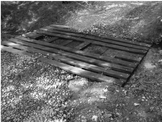
**Figure 4. FORD crossing was reinforced with geotextile, gravel, and mat for a temporary haul road.**
