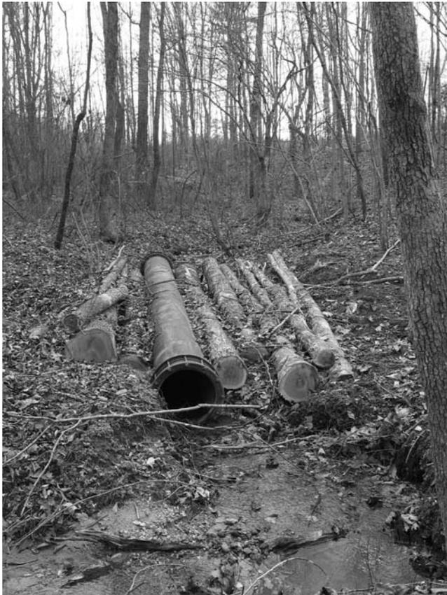
**Figure 3. POLE crossing used a steel pipe and poles for a temporary skid trail stream crossing.**
