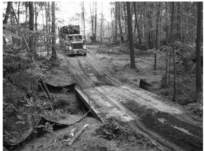
Figure 2. BRIDGE treatment using portable steel panels for a temporary haul road stream crossing.
