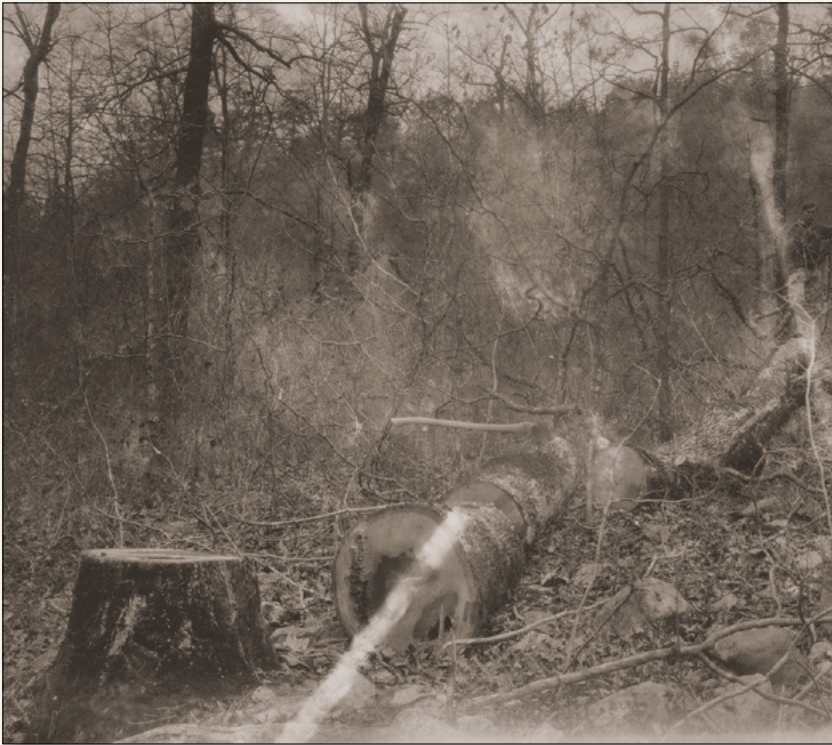
Left: Plate 3. Low utilization of white oak for cooperage. Note rot in the stump cut. The whole tree yielded but one sound bolt. Rock Creek, Mena District, Ouachita National Forest.
