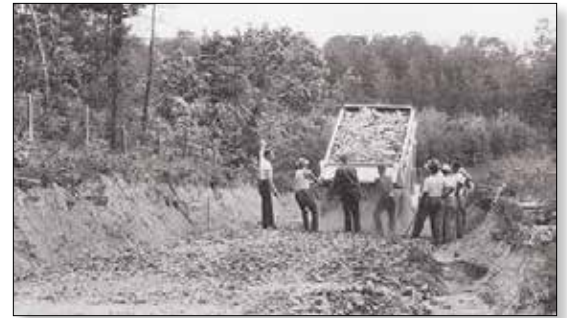
Civilian Conservation Corps crew is applying rock to a newly constructed roadbed.
