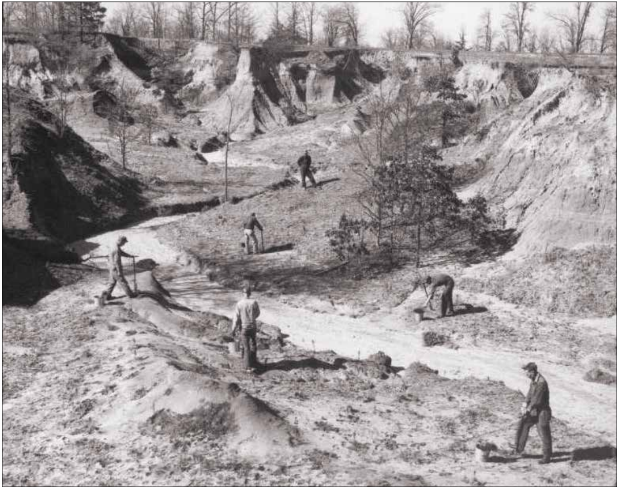
Planting pine seedlings to control erosion was a common practice on severely eroded sites.
