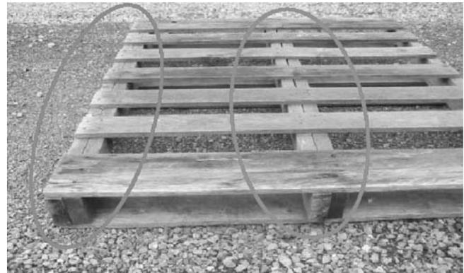
Figure 1. — Example of full companion stringer repairs adjacent to center and outer stringers.
