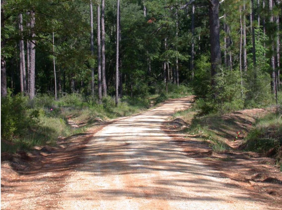
Figure 2. Typical crowned forest road section used in the investigation.
